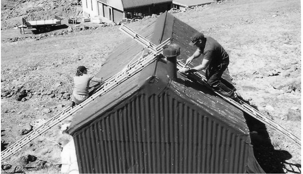
Work on the roof of the RSC's mountain museum Glacier Hut. This shot was taken before the Covid-19 lockdown. Photo: Catherine Gafa.
